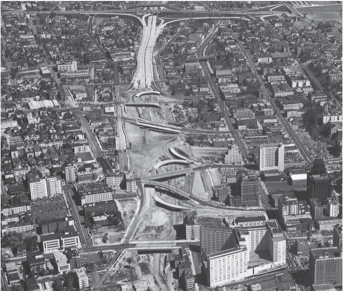
State Route 110 was bulldozed through neighborhoods at the edge of downtown Los Angeles in 1953. (UCLA Geography Aerial Archives.)
