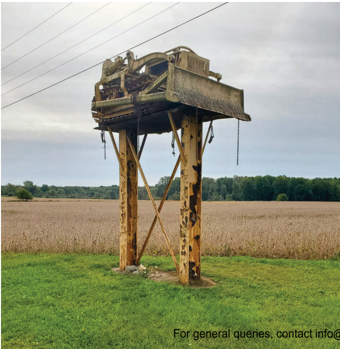
Is demolition the best solution? An exalted excavator above an open field in rural Michigan, 2024. (Amy Hetletvedt)
